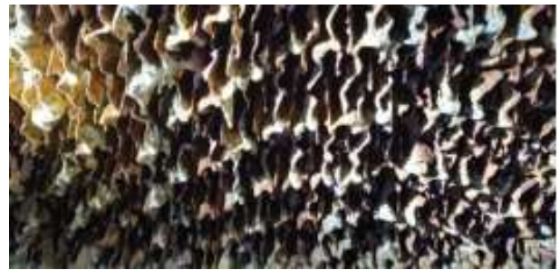
Figure 3. Corrosion and Wear condition of of regenerator in the Low Temperature section.
